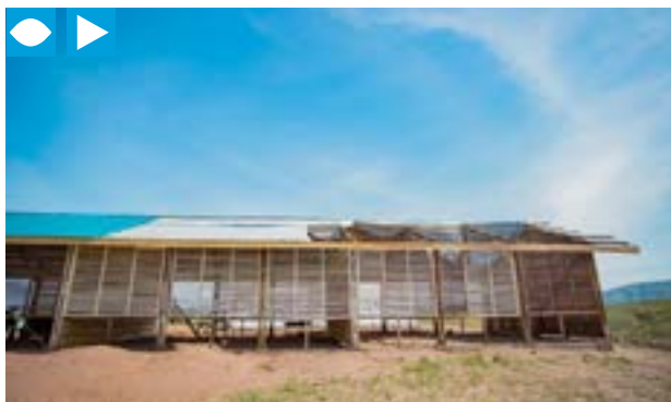
Lubile 1 Primary School in Tanganyika Province, Democratic Republic of the Congo, was destroyed when militia groups clashed and inhabitants deserted the village. Three classrooms made of tarpaulin are being installed with CERF support in February 2021 to allow students to resume classes quickly. UNICEF undertakes the construction of permanent classrooms. | 18 MAY 2021/UNICEF/JOSUÉ MULALA
